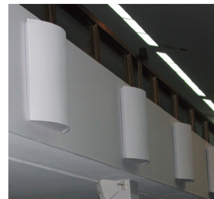
Diffuser panels break up the reflections from the side walls of the Nambour Baptist Church
